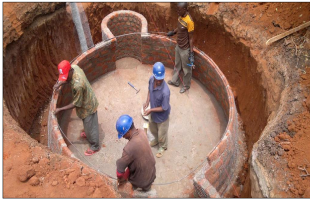
Figure 14 (a): Biogas Plant construction [26]
